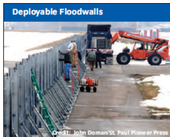
Figure 4: Installation of deployable floodwalls (Source: BNAVC)
