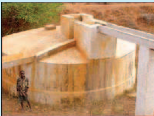
Capture systems help manage water resources more efficiently: Image: Rainwater Storage Tank (Black 2006)
