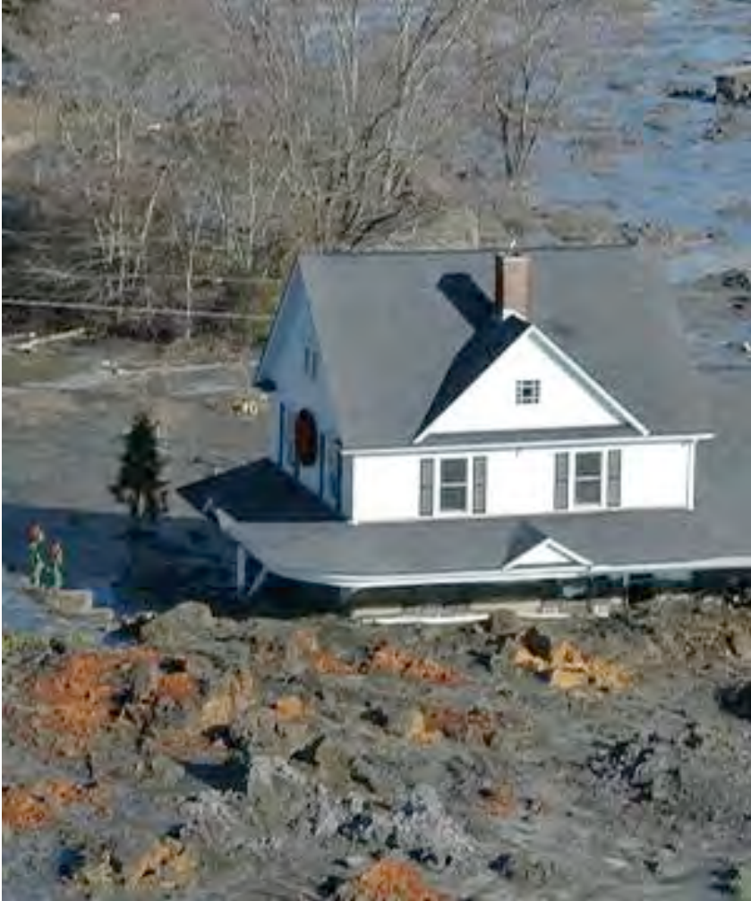
Figure I-3 - Tennessee Coal Dam Failure (Source: KnoxvilleNews, 2008)
