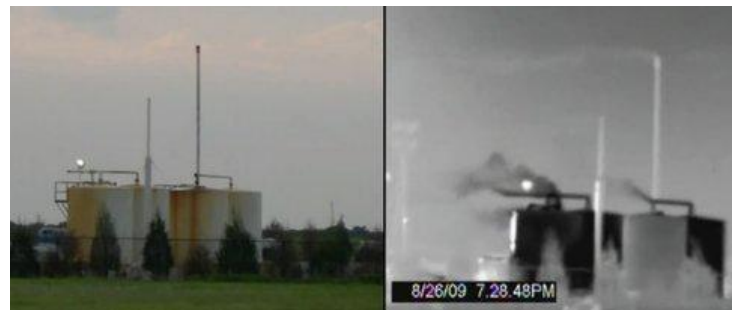
Figure 4.2.3.1 - Methane leakage detection using infrared. The picture on the left shows methane storage tanks taken with a regular camera. The photograph on the right is an infrared (IR) image. The “smoke plumes” are the methane leaks.
