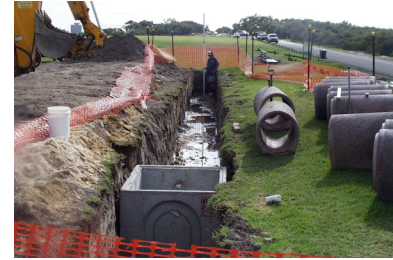
Figure 2.3: Infiltration Trench
