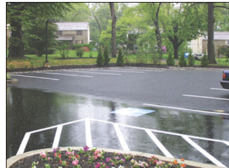
Figure 2.5: Pervious Paved Area
