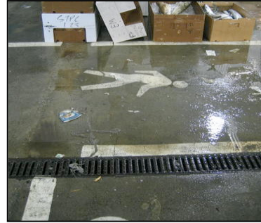
Figure 8: Drains at Fish Market
