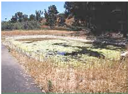
Figure 2.2: Infiltration Basin
